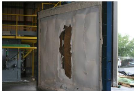
Figure B-8. Exposed Face Immediately Following Fire Test.
