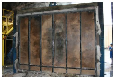
Figure B-10. Condition of Exposed Face Following Hose Stream Test.
